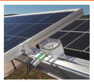
Sensor with polycrystalline cell.
